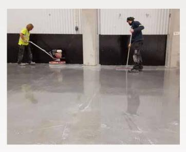
After application Lithurin HARD polish the edges with Edge machine and LC PAD 120/320.
