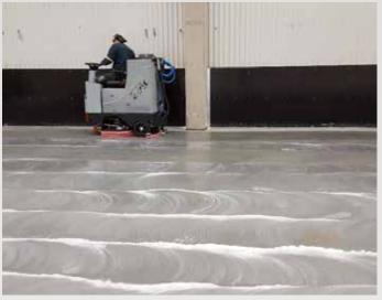
Run with combi scouring round walls with LC Pad 320.
